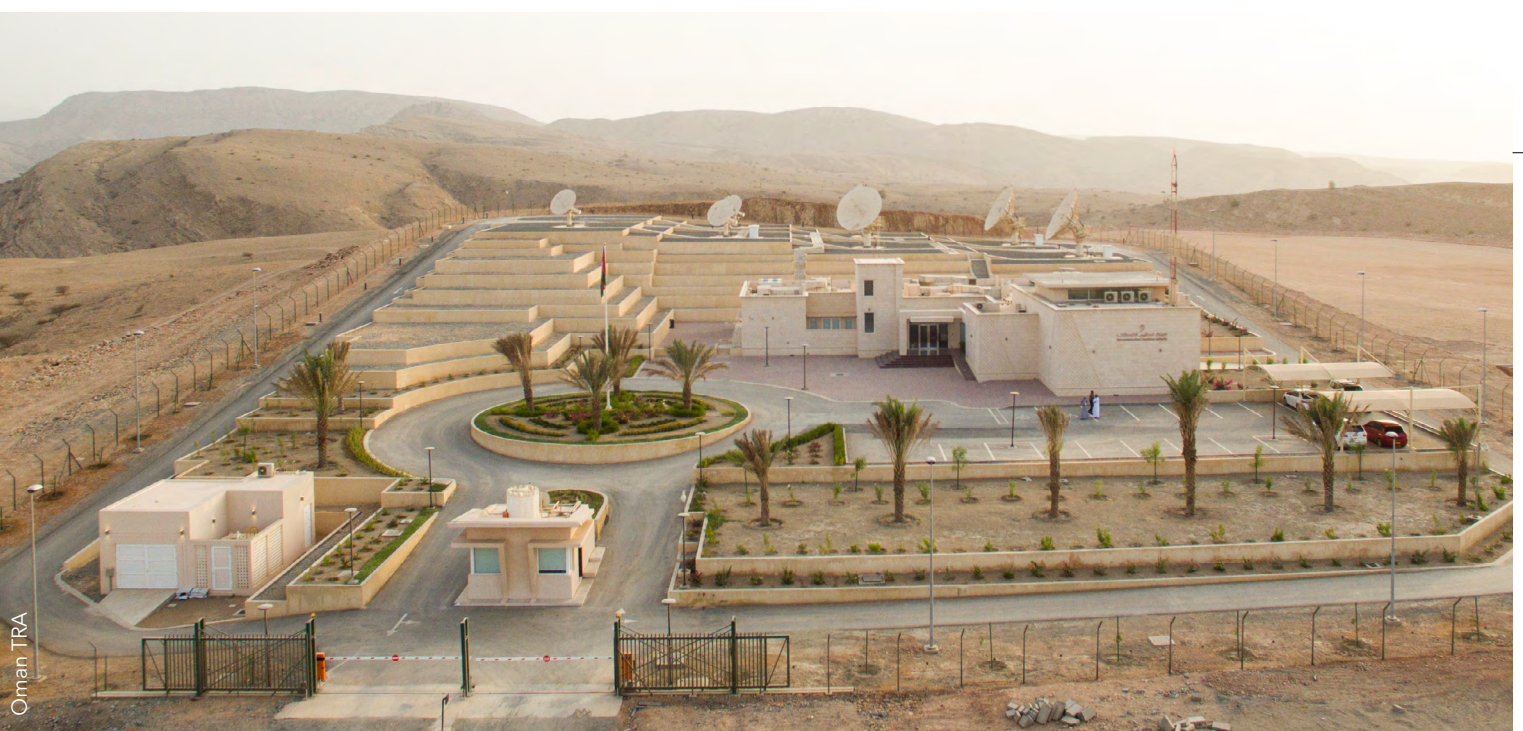
Space Radio Monitoring Station located in Muscat, Oman
